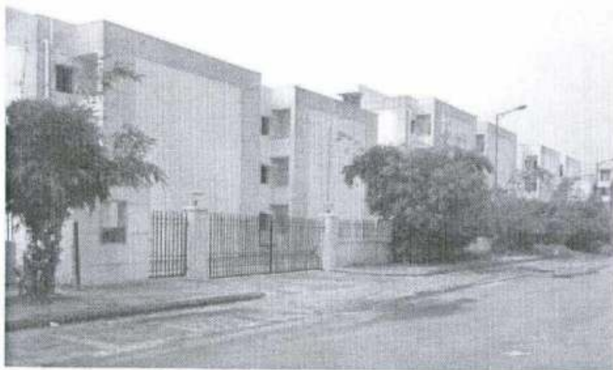
DLF GARDEN CITY, LUCKNOW LIG/EWS -FRONT VIEW
